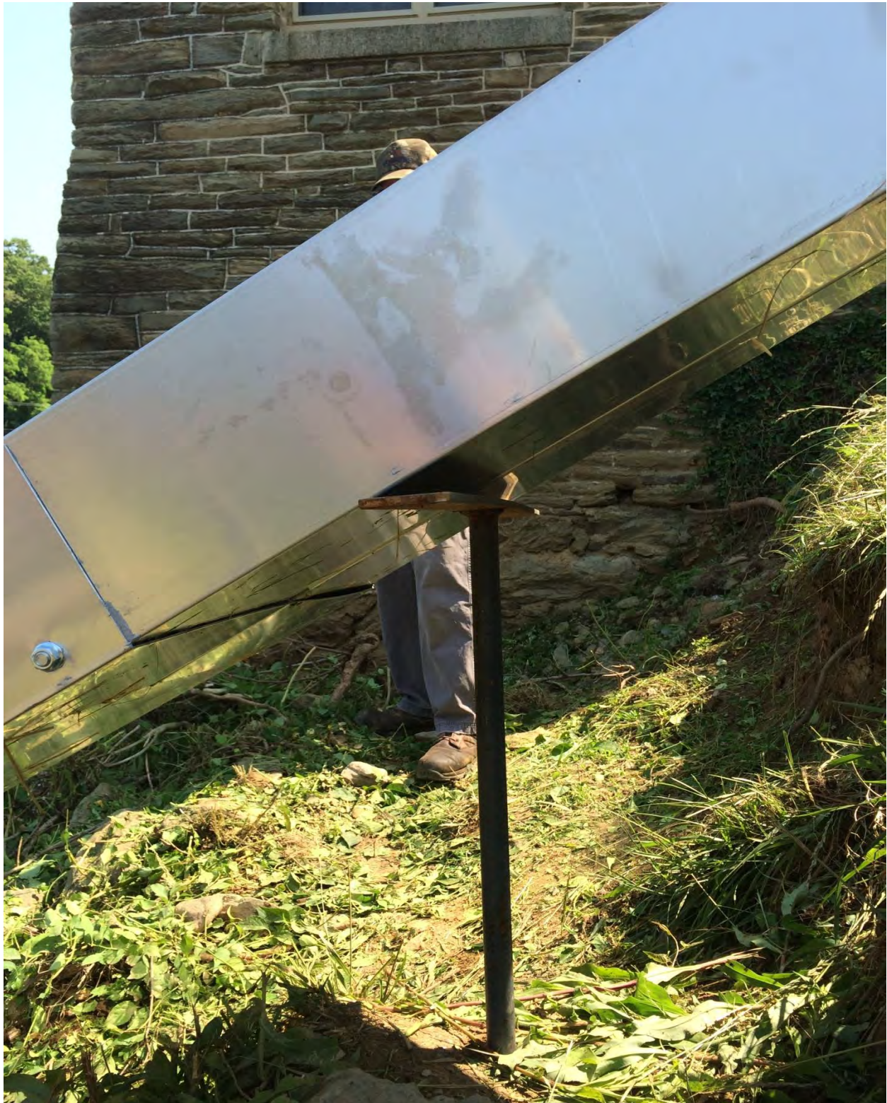
Figure 3.1-2: T-Bar Support for Ramp Support, Octoraro Creek
