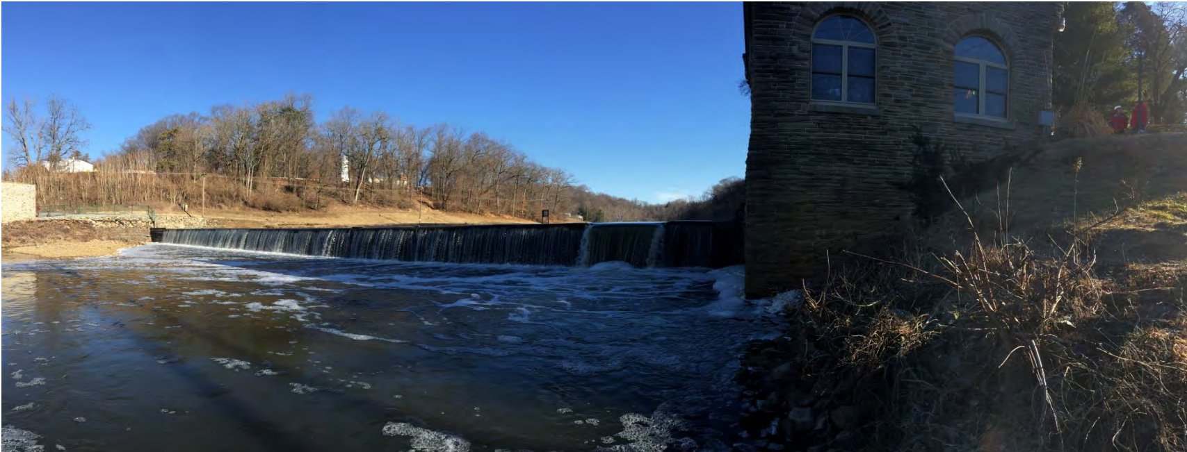
Figure 2.0-2: Location of the Juvenile Eel Collection Facility on South Shore (Left Bank) Of Octoraro Creek Downstream of Art Building
